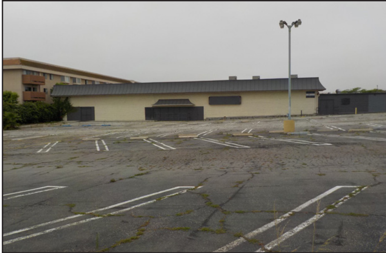
A. Looking west at front of vacant building
