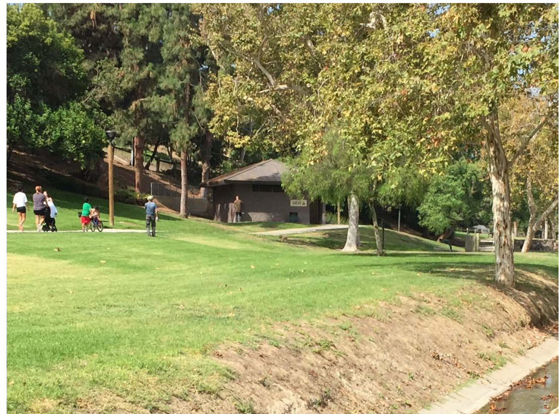
Existing Restroom Facility
