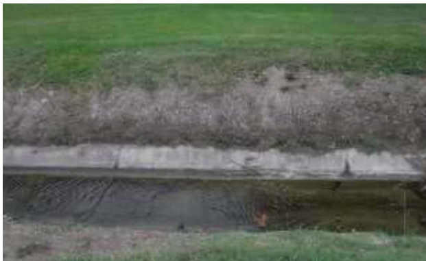
DSCF0024, Creek Channel Soil Profile, Mid-Park, View South
