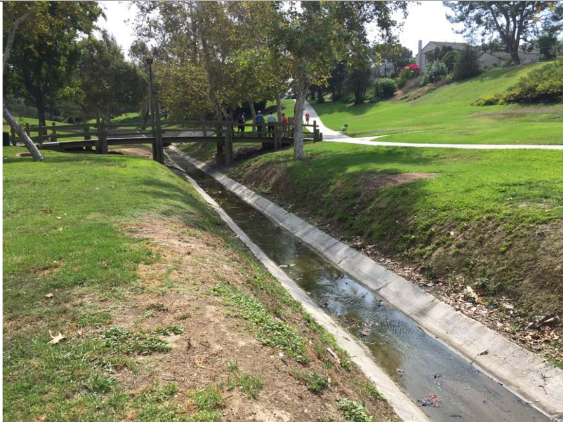
Existing Bridge Crossing
