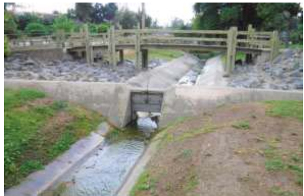
DSCF0035, Check Dam and Foot Bridge, Mid-Park, View West
