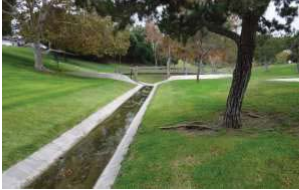
DSCF0003, Overview West, Near Santa Gertrudes Ave.
