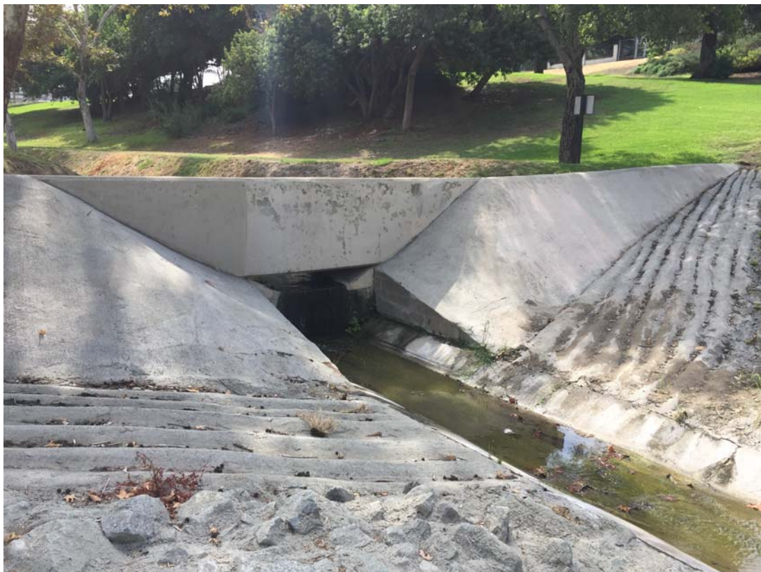
Existing Concrete Check-Dam
