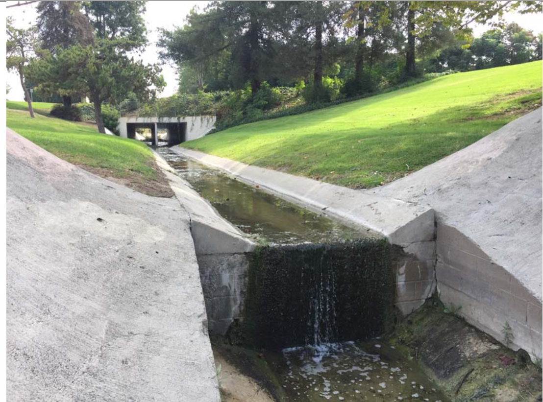
Existing Concrete Channel
