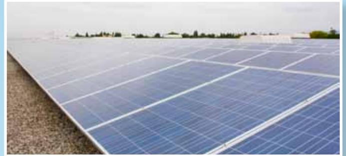
U.S. Foodservice-Los Angeles recently activated a 1.15 megawatt, 4,998 photovoltaic solar panel system on its rooftop, one of the largest solar projects in Southern California. The system is projected to provide 16 percent of the facility's power needs annually.
